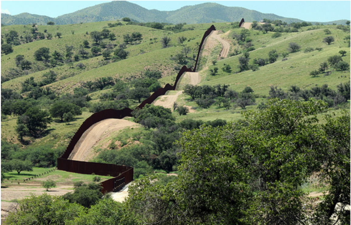
Figure 2: Border Fence at Nogales, Arizona.
